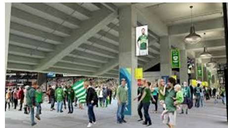
Fig.2: (from left): Superstructure consisting of reinforced concrete moment frames with raker beams and cantilever steel roof truss, raker beams at the seating area connecting to columns
