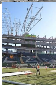
Fig.3: (clockwise from left): Roof truss erection sequence: Truss pieces placed on field for lifting; cranes positioned on both sides of the east wing; a truss piece being erected from the crane on SW 18th Ave side; truss connection to reinforced concrete moment frame and a construction worker doing field adjustments to align truss pieces in position.
