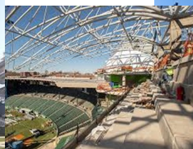
Fig.3: (clockwise from left): Roof truss erection sequence: Truss pieces placed on field for lifting; cranes positioned on both sides of the east wing; a truss piece being erected from the crane on SW 18th Ave side; truss connection to reinforced concrete moment frame and a construction worker doing field adjustments to align truss pieces in position.
