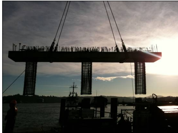
Precast pile bent with rebar cage inserts being lifted into place.
